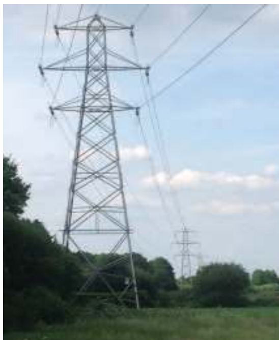
Height Band 2 132kV pylon – Mark Darlow Copyright.
